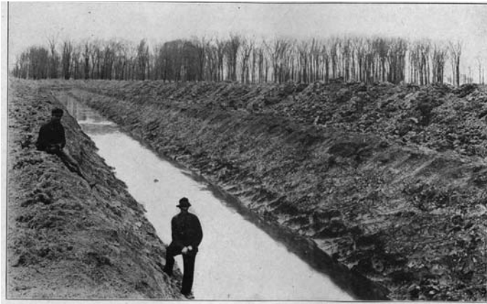
Figure 1.7 1917 Dredging Project in St. Clair County
