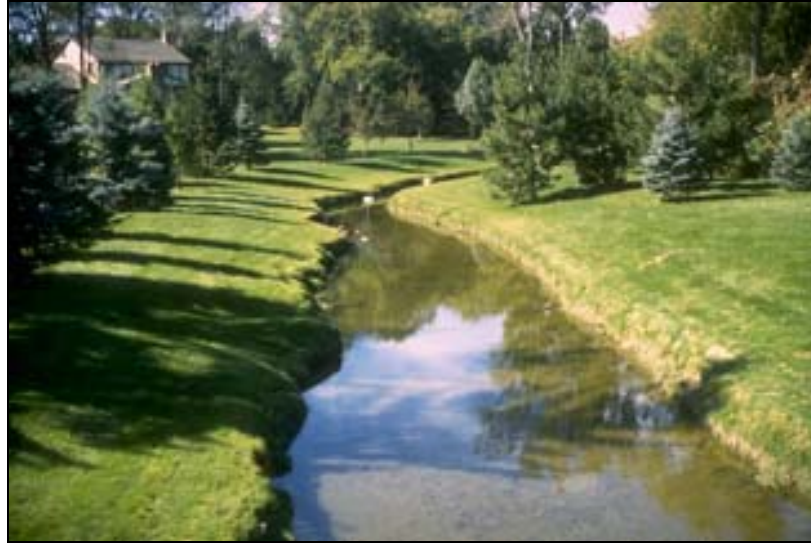
Figure 2.32 Lack of Canopy Cover and Riparian Buffer in Urbanized Area
