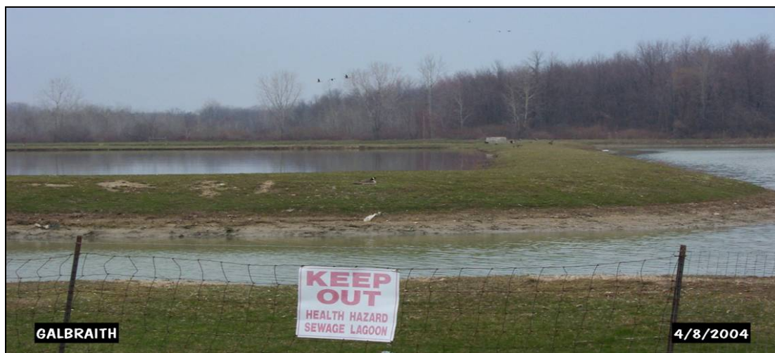
Figure 2.22 Sewage Lagoon that Discharges to Galbraith Drain in the LHD Subwatershed
