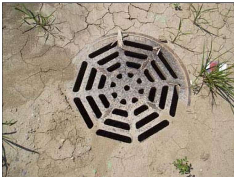
Figure 2.16 Sediment Pathway to Surface Water through Stormwater Conveyance System
