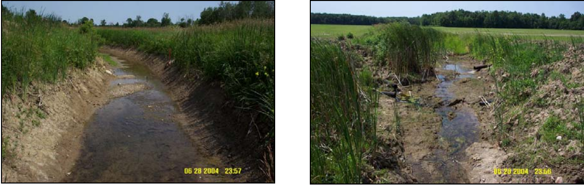
Figure 2.5 Hydromodifications such as Ditching and Tile Drainage in Agricultural Areas Impact Watershed Hydrology by Increasing Stormwater Runoff Quantities and Decreasing Groundwater Recharge and Baseflows in Streams (photos taken at Norman Road along Thomas Drain in the LBR subwatershed)
