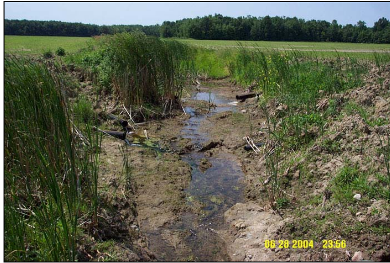
Figure 2.30 Tile Drainage into Thomas Drain with Erosion and Nutrient Inputs
