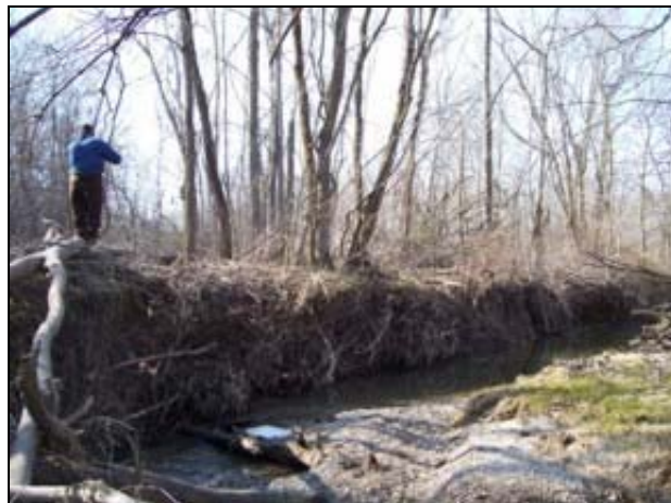
Figure 2.19 Streambank Erosion along Burtch Creek in the LHD Subwatershed
