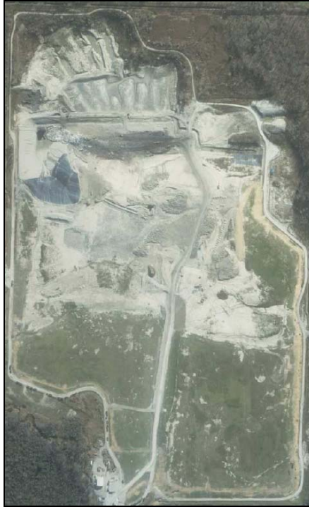
Figure 2.15 Aerial View of Smiths Creek Landfill in Kimball Township
